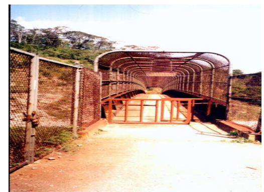
LHT Bridge over I76.
